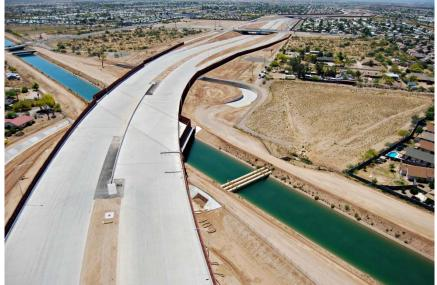
utility relocation. The uniquely engineered straddle substructure made it possible to economically bridge an arterial roadway and the CAP canal at a difficult angle. The bridge is the first of its kind in Arizona. The project cost savings allowed the inclusion of a fourth general use lane each way. Congratulations Stanley Consultants Inc. for delivering this exceptional engineering project under budget and ahead of schedule!!!
